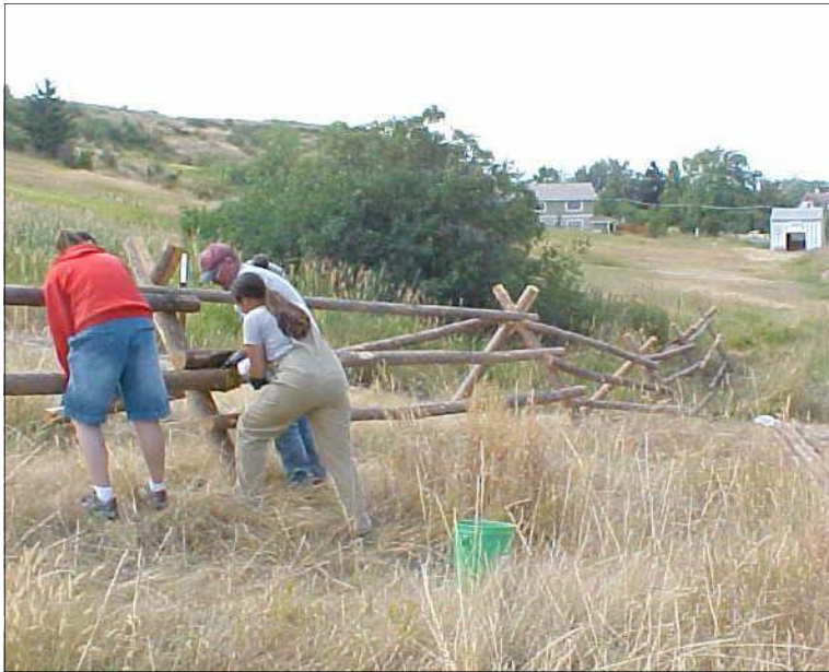
Campus Corps members participate in a fence-building service project.
